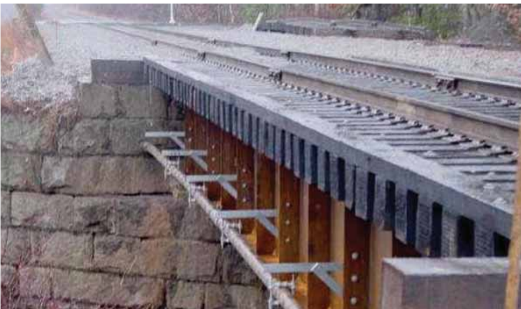
New Bridge at Bellamy River Photo by Phil Corder
