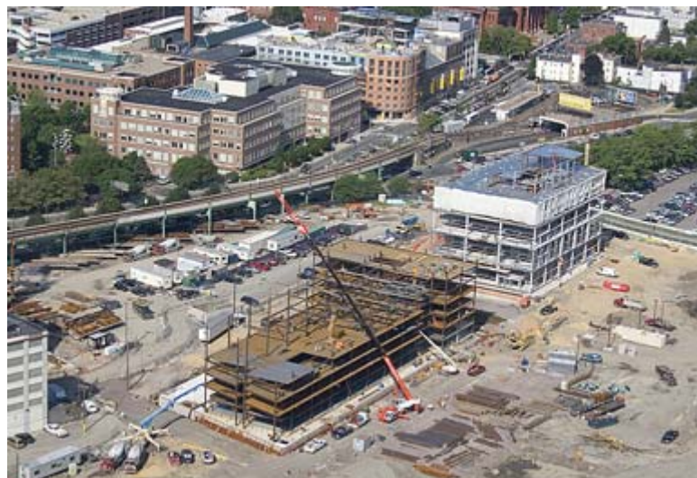
Aerial View Photographer: Mark Flannery Photography (8/3/06)
