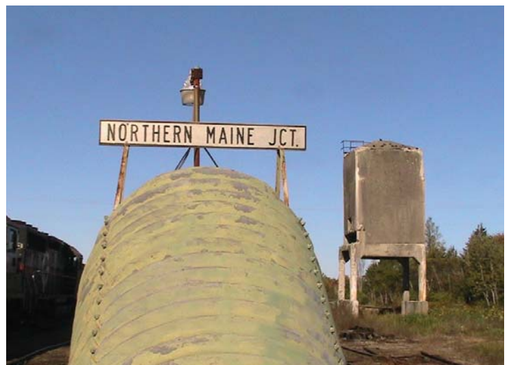
Station sign on former subway to cross under tracks Photo by Dwyann Williams
