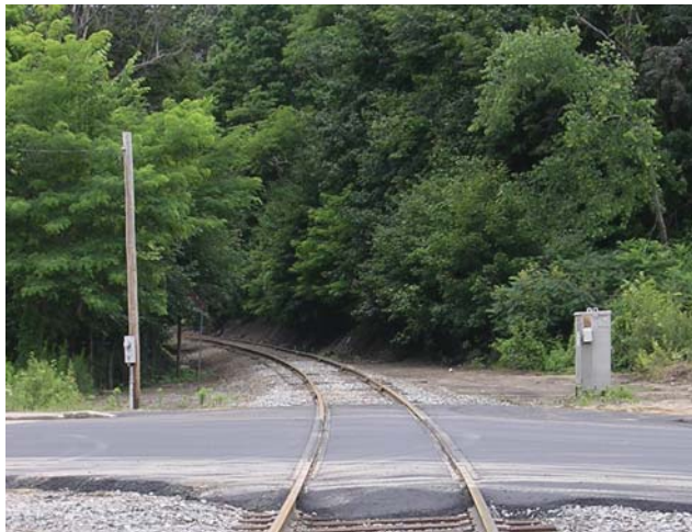
Depot Street - AFTER Photo by: R.A. Blanchard
