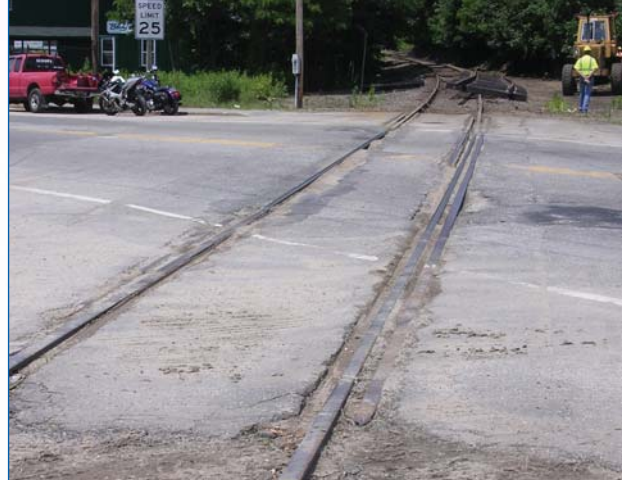
Depot Street - BEFORE Photo by: R.A. Blanchard
