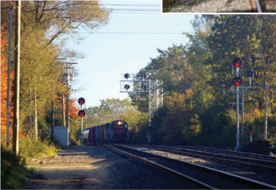
Completed Interlocking at Dover, NH
